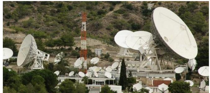
Makarios Teleport hosts a large number of earth stations that provide links to numerous satellites, supporting Cyta's extensive satellite telecommunications network. There are transmit antennas operating in most satellite frequency bands, such as C, S, Ku standard and extended, DBS and Ka band. In addition, the Teleport offers extensive reception capabilities with a large antenna farm deployed to receive content from the main satellites visible from Cyprus.
